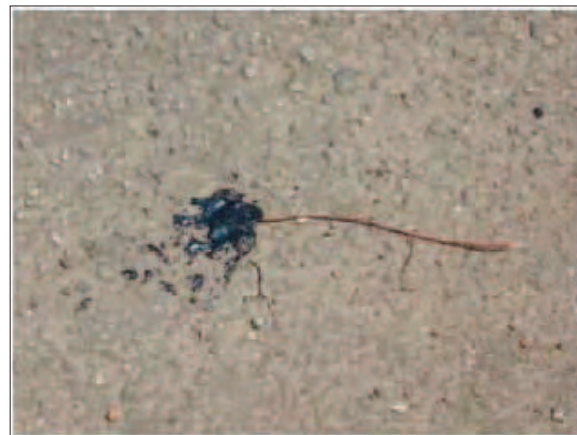
Figure 3: Thermocouple installed in the pavement
