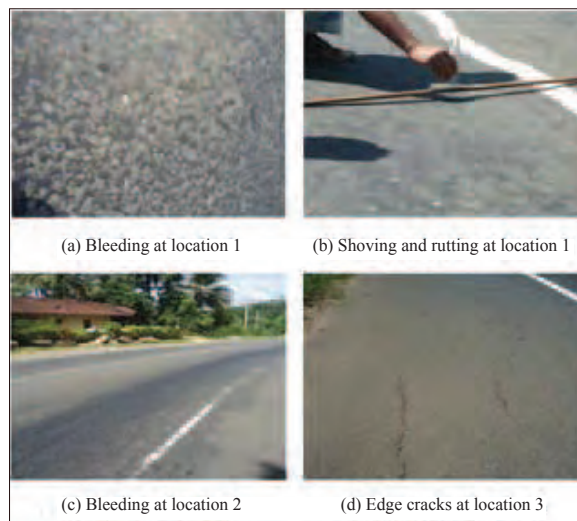
Figure 4: Pavement distresses
